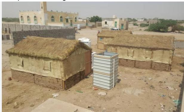
**A Transitional Shelter Unit (TSU) is built with iron pipes and local materials.** It withstands extreme weather conditions, such as heavy rain, strong wind, humidity and heat. This longer-term shelter solution can last up to five years with proper maintenance.
