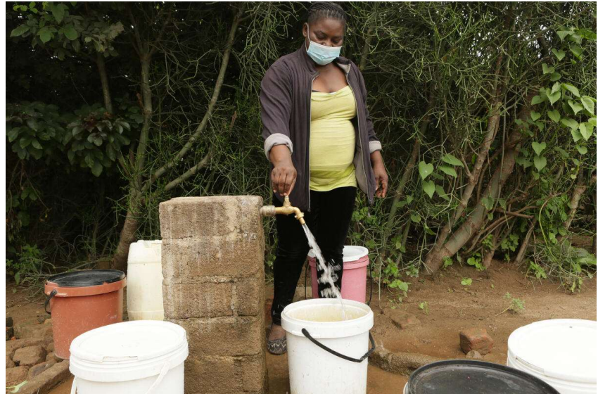
A refugee from the DRC turns on a tap at Tongogara refugee camp, Zimbabwe, which is part of the newly improved water system. Improved access to water helps to promote good hygiene practices to prevent the spread of COVID-19 ©UNHCR/ Tsvangirayi Mukwazhi
