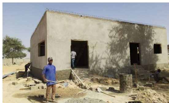
The preventive care unit of the new health center of Chadakori is under construction
