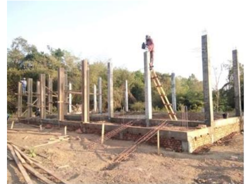
Ongoing construction of primary school in Kayin State. Photo: UNHCR
