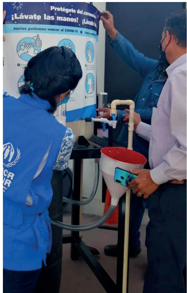
Handwashing installation at DIF facilities, San Luis Potosí, San Luis Potosí.
