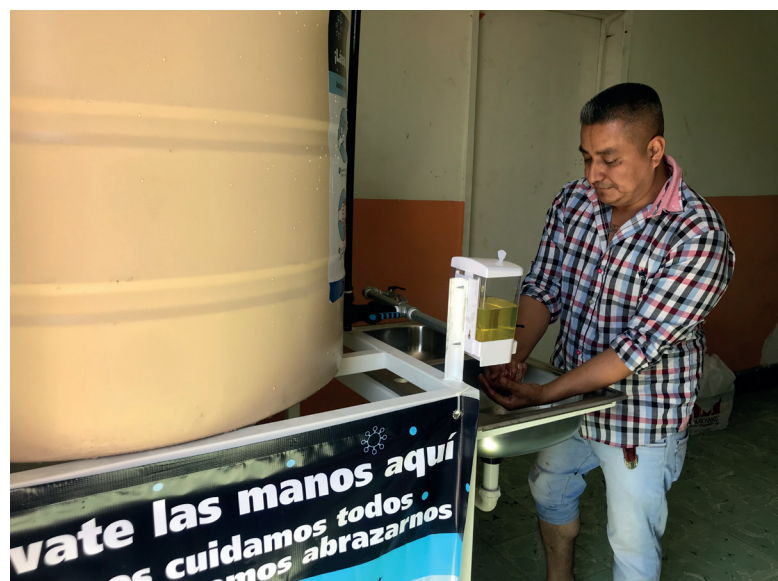
Handwashing installation at DIF facilities, León, Guanajuato.
