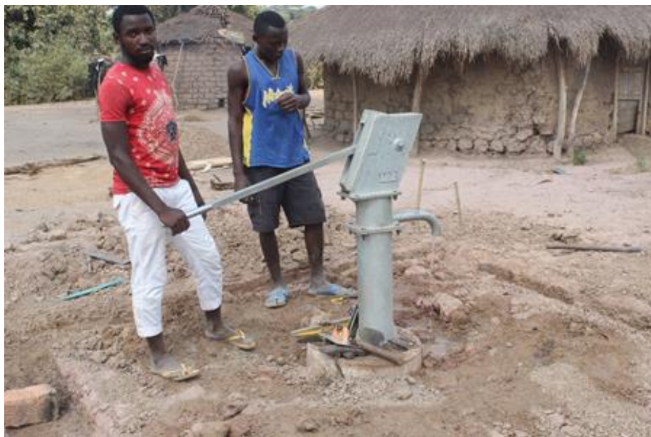
New borehole equipped with a manual water pump in Yakoma (Nord Ubangi) © UNHCR/G. Nentobo
