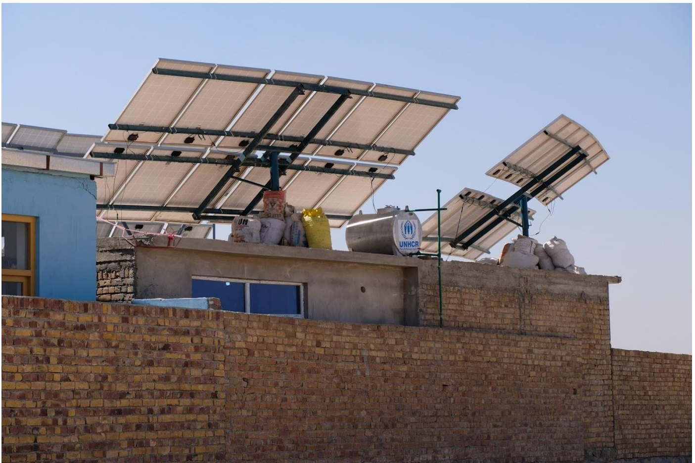
A UNHCR-constructed school in Tarakhail Daag, a priority area for return and reintegration in Kabul province, uses solar panels for electricity and water. UNHCR/H.Macdonald
