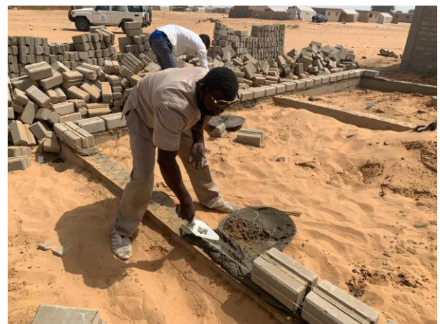
Construction of durable houses in Diffa © Ramatou Issa
