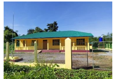
Before and after: Construction of a primary school in Kayin State. Photo: UNHCR
