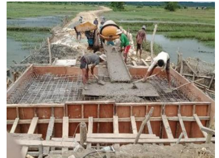
Village access road improvement, Rakhine State Photo: UNHCR
