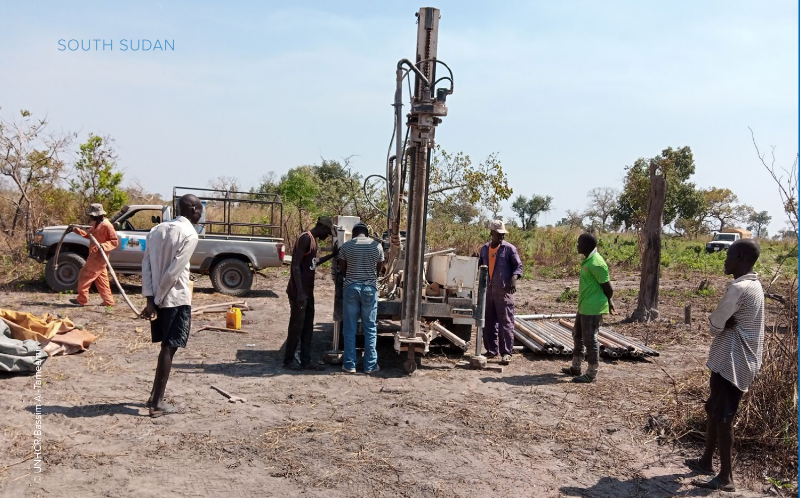
Drilling of borehole in Western Bahr Ghaza.
