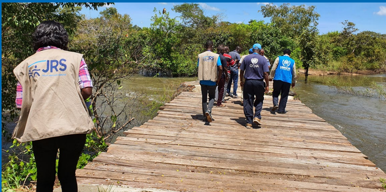
Sue bridge after rehabilitation.
