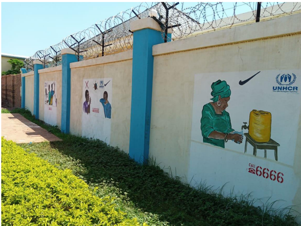
South Sudan. Youth from internally displaced and host communities have renovated the external walls of the UNHCR office to reach out to people with hearing impairments.
