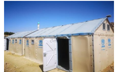
UNHCR installed two RHUs for use as temporary classrooms for girls attending grades 1-3, who otherwise would have missed school due to distance. © UNHCR/ Damien McSweeney.
