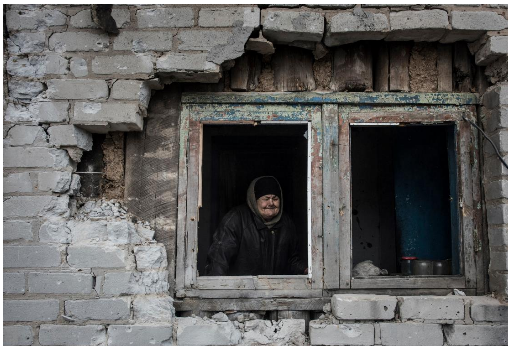
An elderly woman looks through the window of her house, badly damaged by shelling in Avdiivka, Donetsk region. A surge of violence in eastern Ukraine in late January 2017 left a small town of Avdiivka in Donetsk region and its 22,000 residents without electricity, heating and water for a week amid harsh winter condition. Fierce fighting has damaged critical infrastructure and destroyed the homes of nearly 200 families. UNHCR supported a government-led response by delivering 40 tonnes of humanitarian assistance for 2,000 people, including emergency shelter materials and relief items such as of blankets, bedding and towel sets, jerry cans, buckets and winter clothing. Photo: UNHCR Ukraine/Evgeny Maloletka
