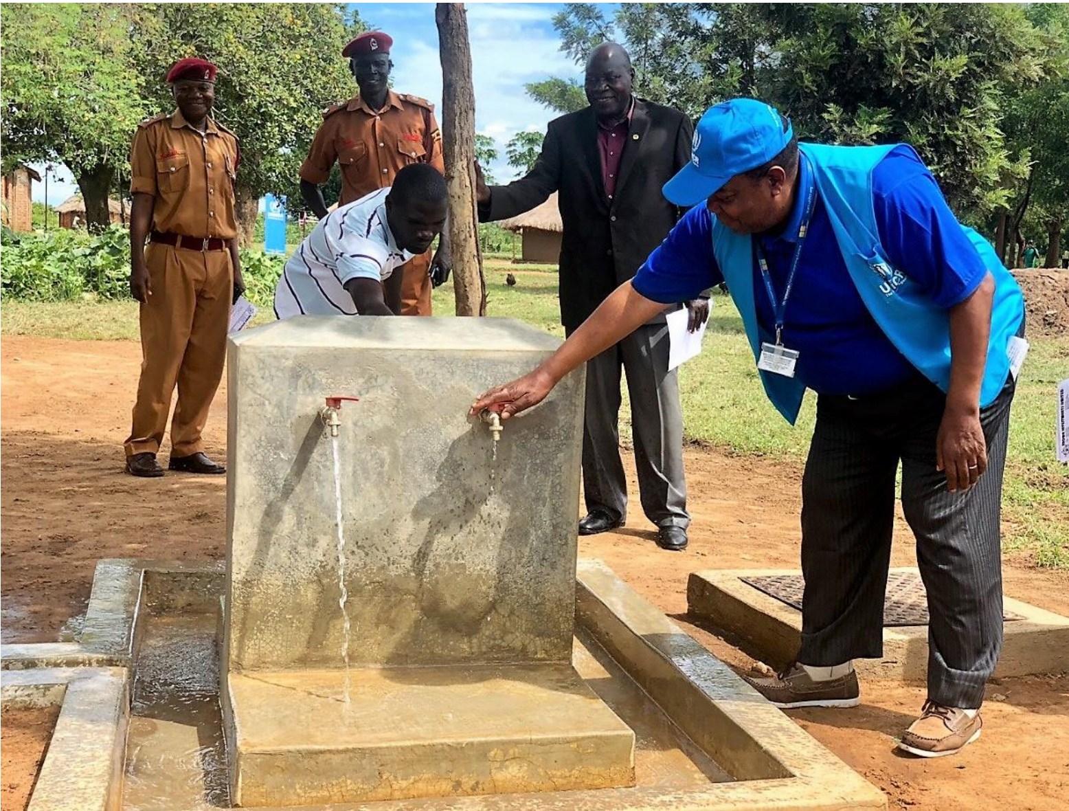
UNHCR and local authorities inspect the upgraded water system of Olia Prison in Adjumani (UNHCR/ M. Charles)
