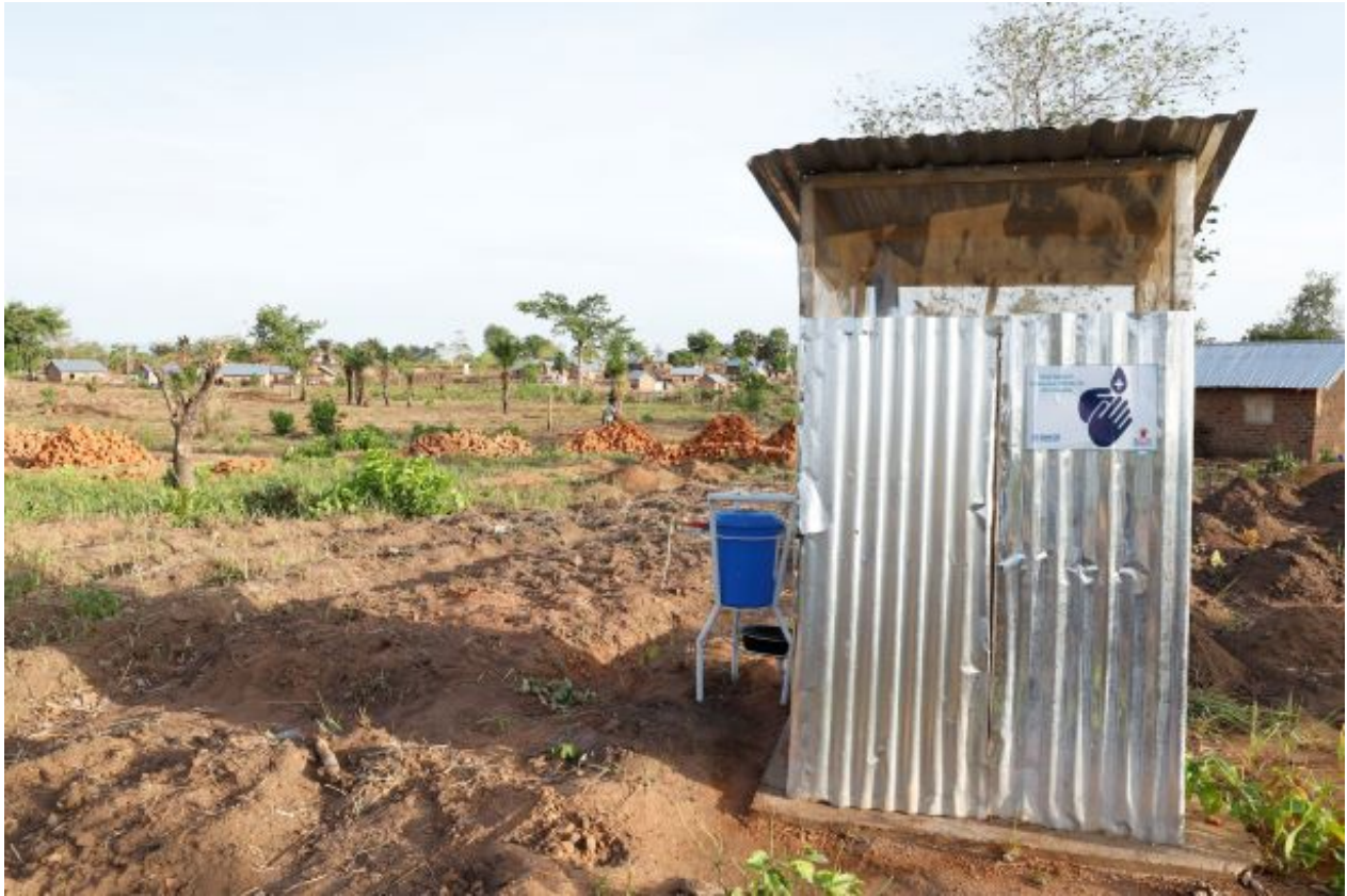
Additional sanitation facilities (toilets, bathrooms) are being added to improve hygiene conditions in the refugee settlements. Handwash station and toilet in Ukende settlement, Ogoja LGA, Cross River State, 08 April 2020. ©UNHCR/Tony Aseh
