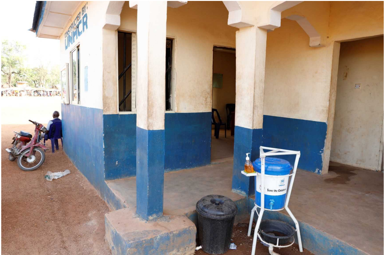
The Cross River State Emergency Management Agency's office in Adagom refugee settlement, Ogoja LGA, has a handwashing station with water and soap for all refugees seeking assistance from the office. 08 April 2020. ©UNHCR/Tony Asch
