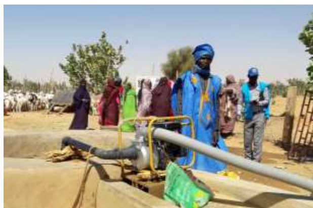
UNHCR supported the improvement of a water pumping system for the community of Lemghayse village, in the Bassikounou area.
