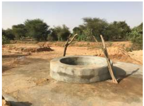
A new water point for the host community in Boulingala, a village in the Bassikounou region. ©UNHCR/José M. Cáceres 2017
