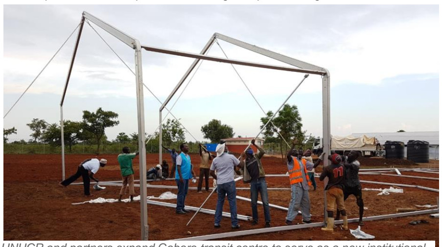
UNHCR and partners expand Goboro transit centre to serve as a new institutional quarantine facility in Uganda's Yumbe district. © UNHCR/O. Nasibov.
