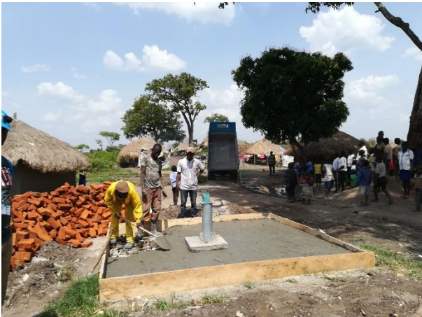
Borehole construction at Biringi settlement © UNHCR/Lopes
