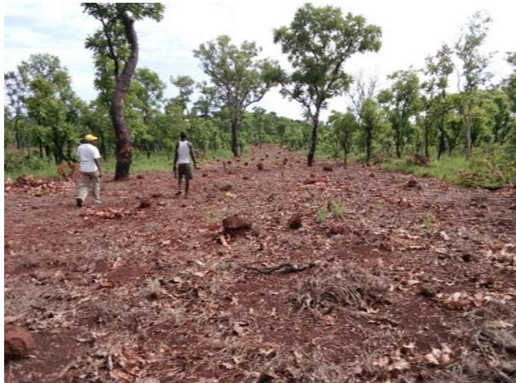
Clearing of the area where transitional shelters for refugees in Ndu will be constructed, Bondo Territory, Bas-Uele Province © UNHCR/N. Gergely
