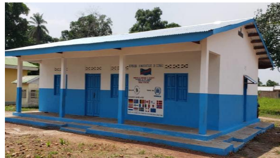
New registration office constructed by UNHCR in Libenge, Sud Ubangi Province. © UNHCR/G. Nentobo
