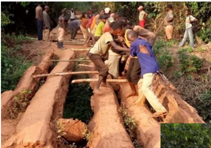
Rehabilitation of a bridge along the road between Monga and Ndu, Bondo Territory, Bas –Uele Province © UNHCR/G. Nentobo
