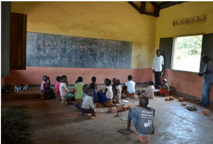
Primary school of Kaka site before and after rehabilitation © UNHCR/A. Cadonau/M. Masimango
