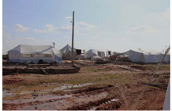
Muddy ground in an IDP site in Idleb negatively affected tents installation © Maram Foundation
