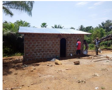
Completed shelter in Boko @UNHCR Guiglo
