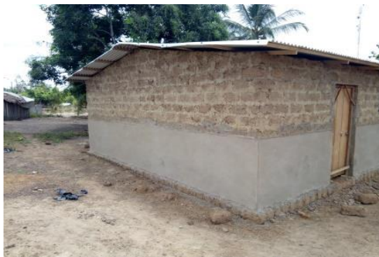
Completed shelter in Bakoubly @UNHCR Guiglo
