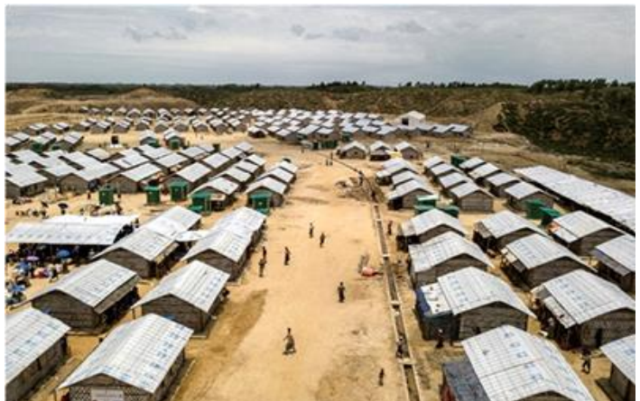
An aerial view of Camp 4 Extension shows shelters and drainage system built after proper site planning. © UNHCR/Adam Dean
