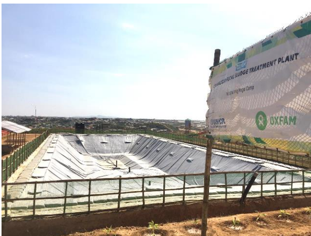
UNHCR and partner OXFAM have established the first large-sized fecal sludge treatment plant in Kutupalong refugee settlement. It's also the first time the specific technology of using covered lagoons is used in Bangladesh. ©UNHCR/S. O'Brien
