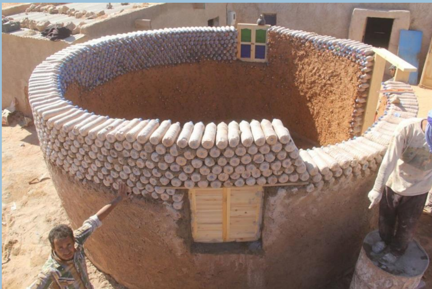
A young Sahrawi refugee builds a weather-resistant shelter out of recycled plastic bottles filled with sand at a camp in Tindouf, Algeria. © UNHCR
