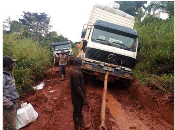
The severely damaged road to Bele, Haut Uele Province. © UNHCR
