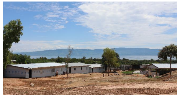
Rehabilitated dormitories at Mongemonge Transit Center, South Kivu. © UNHCR/Sanne Biesmans
