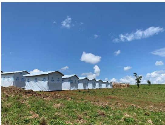
Shelter construction in Ddrodro, Djugu Territory. © UNHCR/Anja Pirjevec
